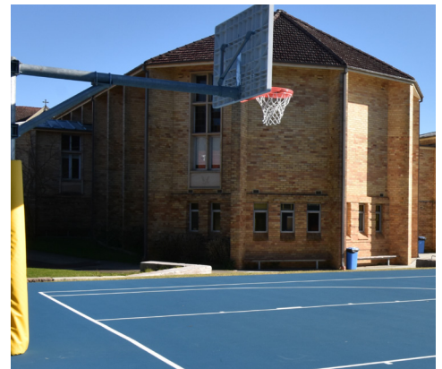
Brick fin buttresses and cream coloured brick finish to the Library
